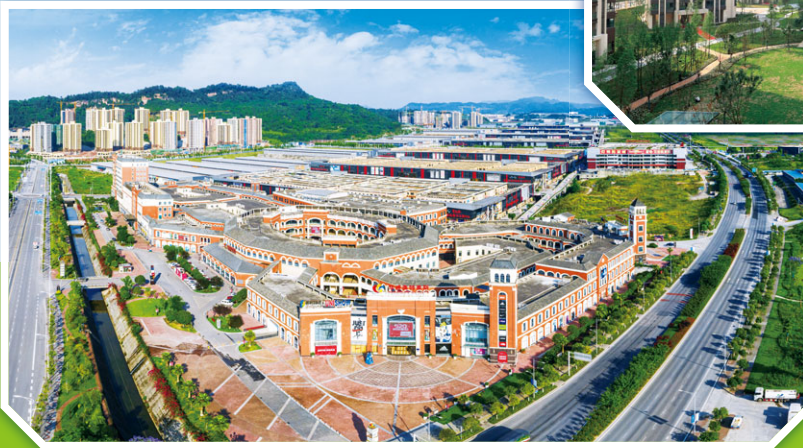
Huasheng Outlet and International Hardware Materials and Machinery Products Expo and Trade Centre in CSC Chongqing 重慶華南城的華盛奧特萊斯廣場及國際五金機電展示交易中心
